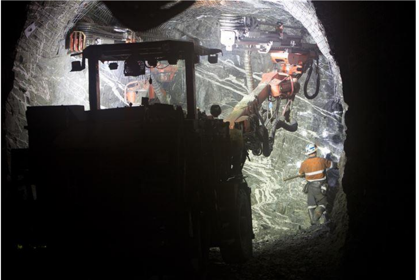
Figure 5. Jumbo mechanised Development immediately adjacent to the old 14 Level North of the A1 Gold Mine.
