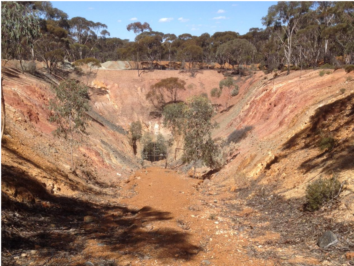
Figure 3: 5B box cut and portal entrance to the decline
