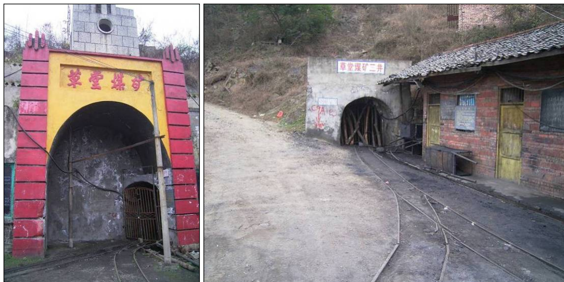
Plate 1: Caotang Pit No1 Portal (L) and Pit No2 Portal (R).
