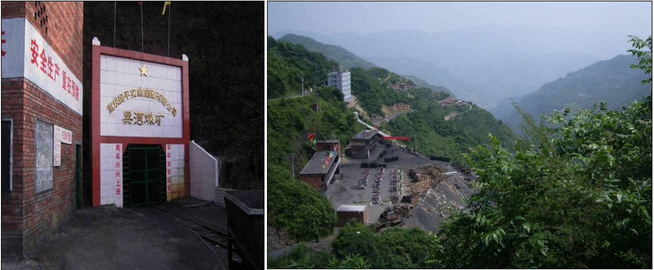
Plate 2: Heiwan Mine Pit No. 1 (L) and View South Over Pit No1 Main Portal towards Main Road and New Office (R).
