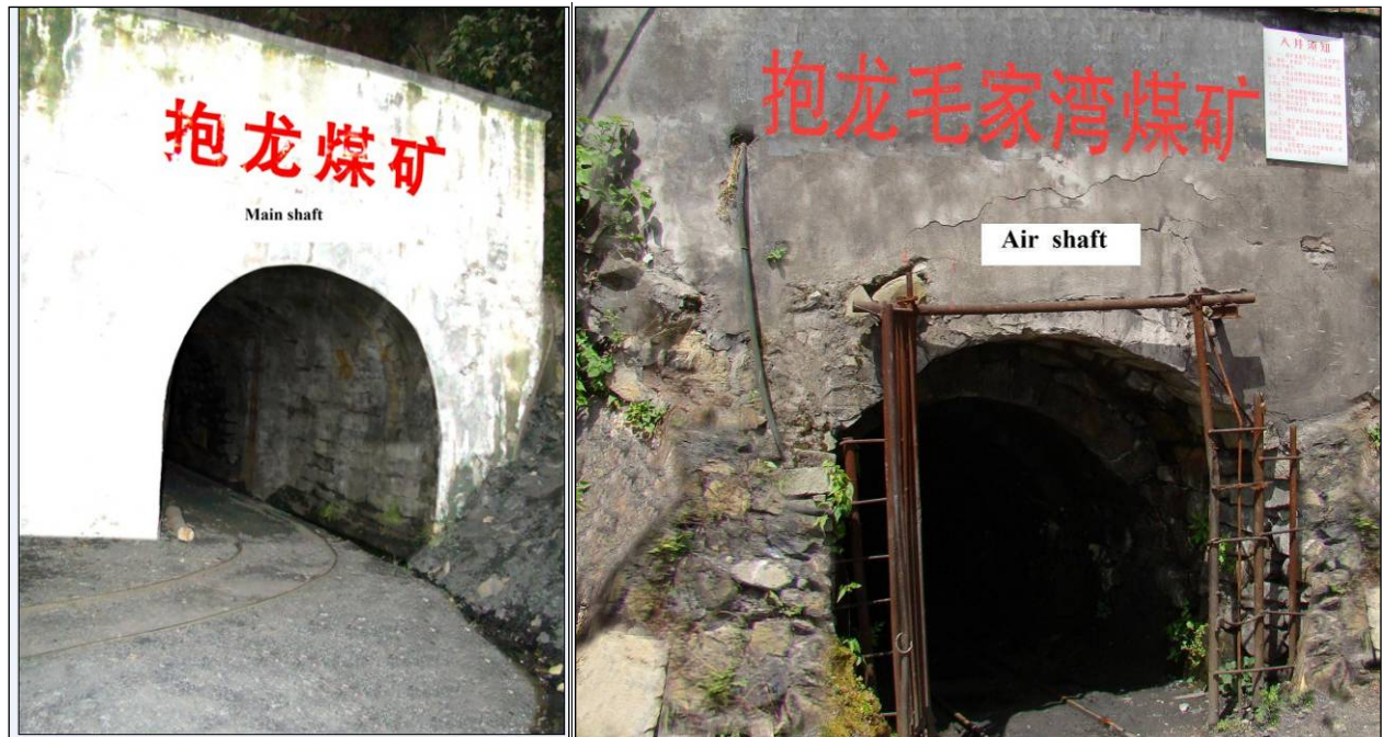
Plate 3: Baolong Maojiawan No 1 East Mine Production Adit (L) and Ventilation Adit (R).
