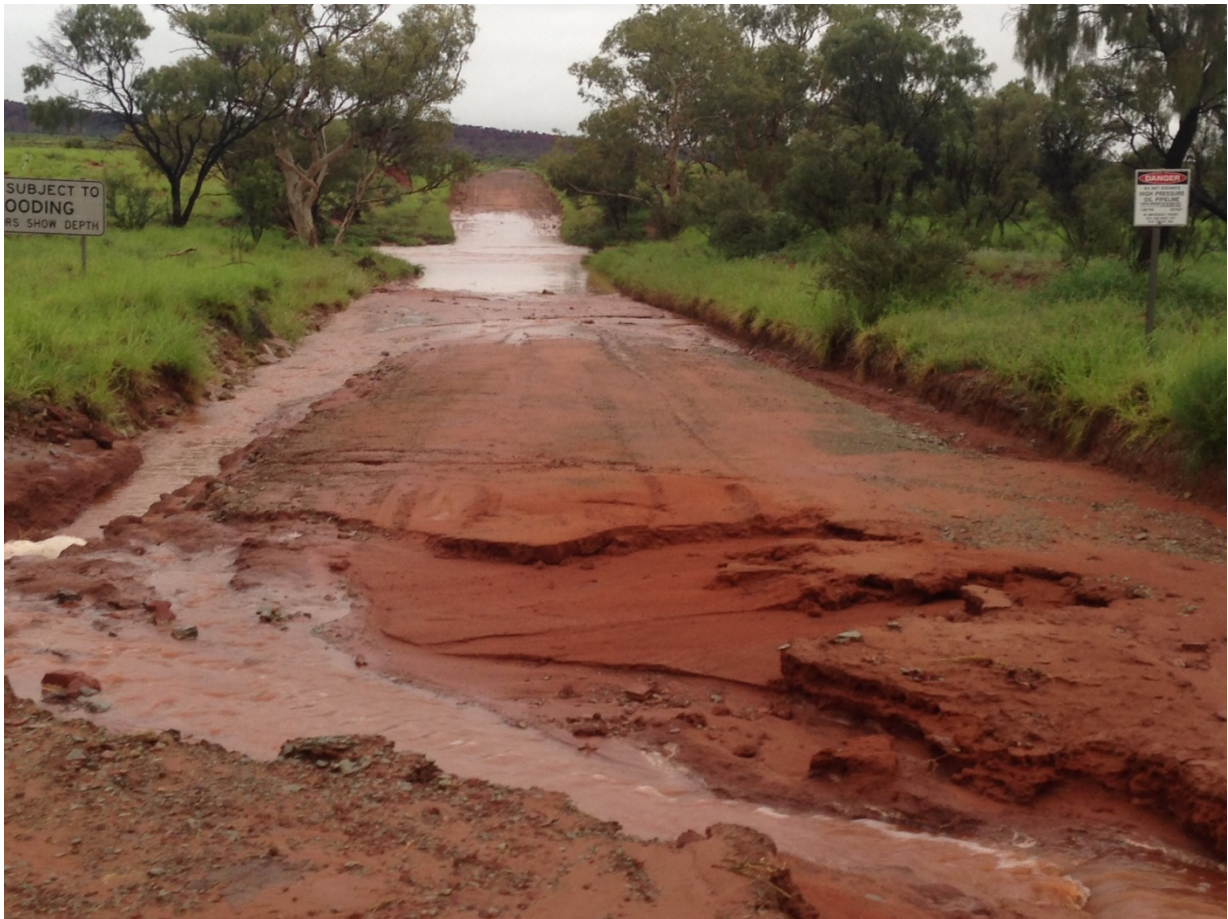
Figure 2: Roads across all fields were affected by wash-outs and flooding, resulting in road closures.
