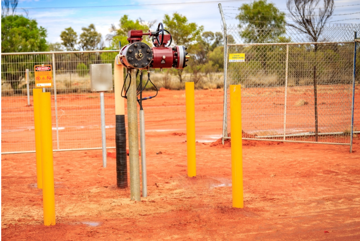
Figure 5: Future connection for Central to deliver gas into the Palm Valley-Alice Springs pipeline is now in place at BECGS compound.
