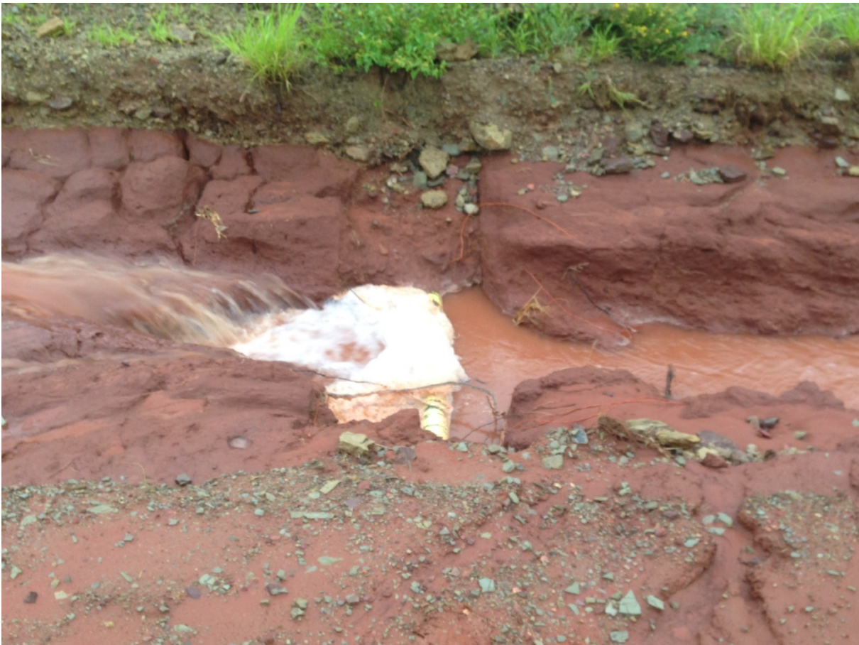
Figure 4: Roads have required multiple repairs after frequent major rain events.
