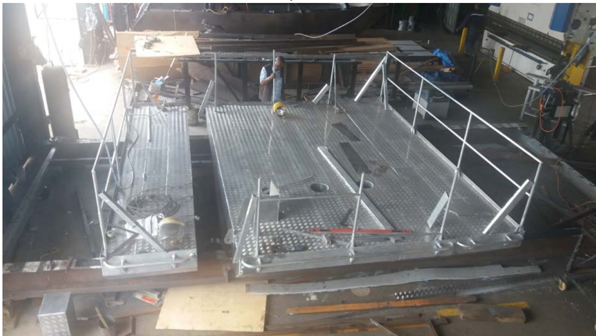
Sonic drill rig barge platform being inspected by Amex marine consultant Mr Matai Baleimatuku
