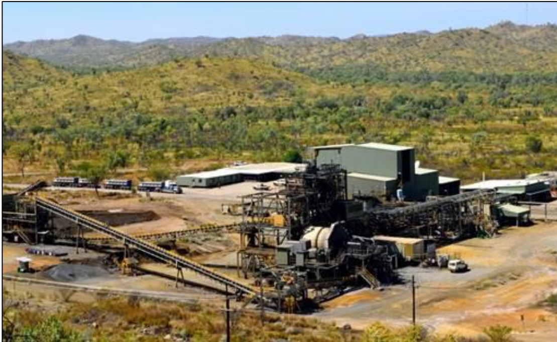
Figure 9 – Savannah Processing Plant
