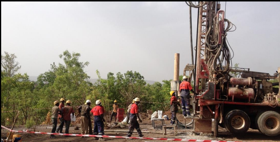
READILY ACCESSIBLE DRILL RIGS AND EQUIPMENT
