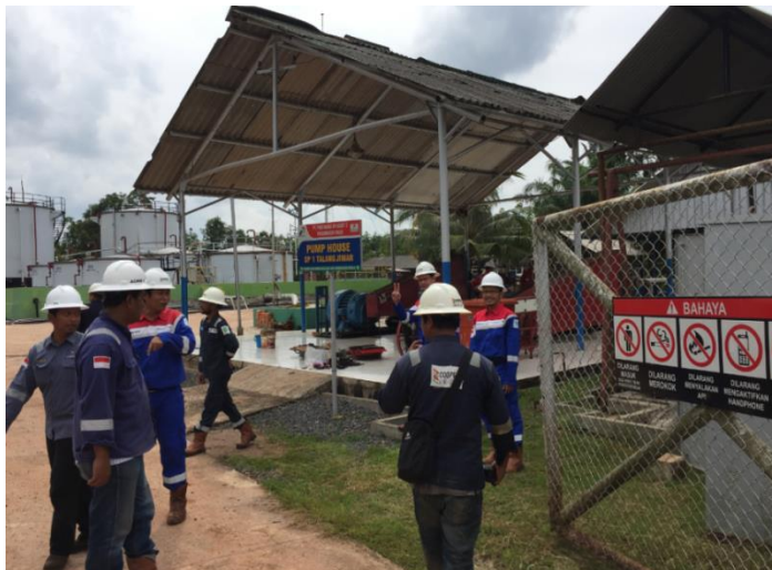
Ground crew at Talang Jimur pump station
