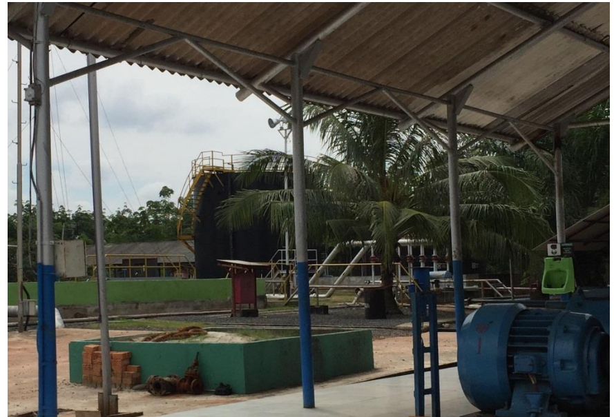
Talang Jimur Transfer Station
