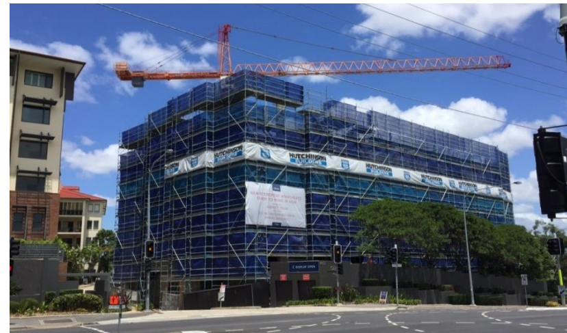
Clayfield construction site
