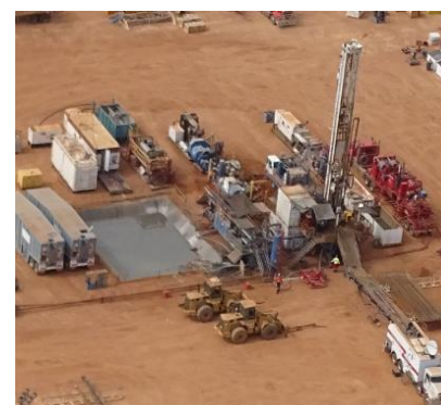
Tubridgi gas drilling rig
