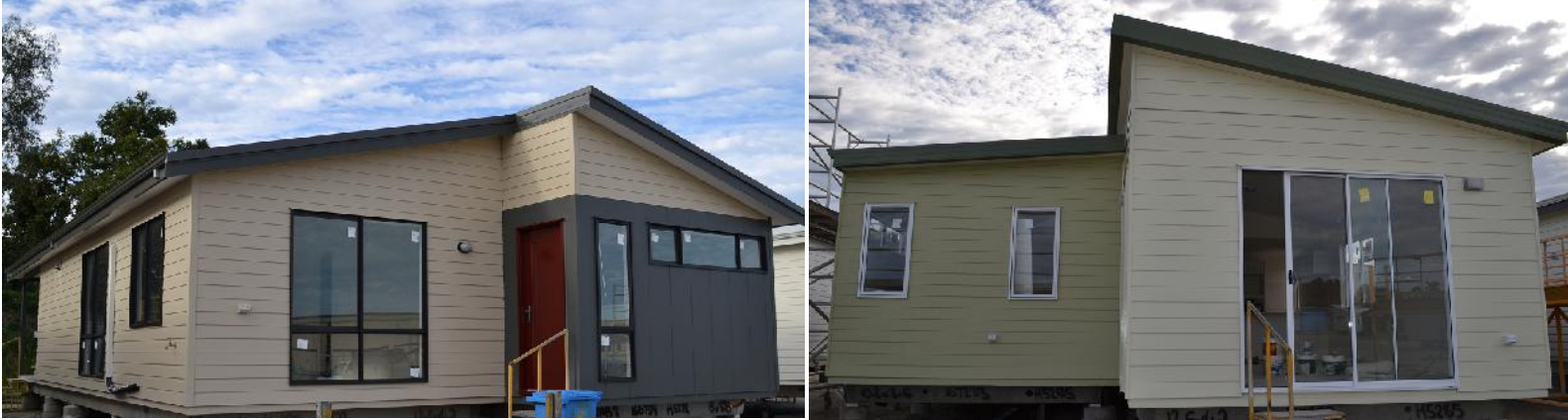
Homes under construction for National Lifestyle Villages, Western Australia
