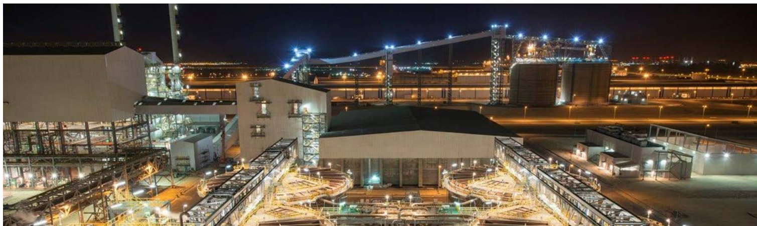
Ma'aden Alumina Refinery, Saudi Arabia
