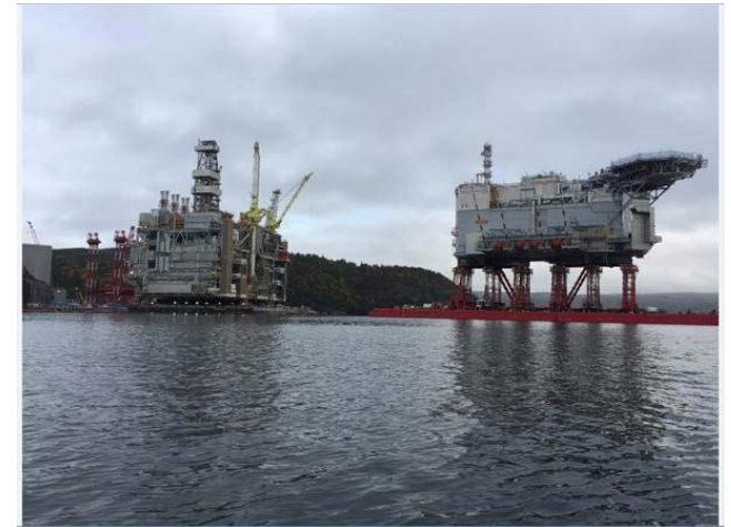
Installation of the accommodation module on the Hebron topsides, Bull Arm, Newfoundland and Labrador (NL)
