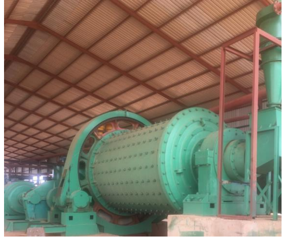
Kipushi Processing Plant - Flotation Cells and Ball Mill
