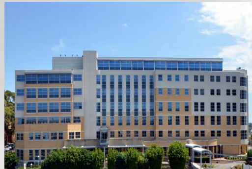
New accommodation wing at North Shore Private Hospital
