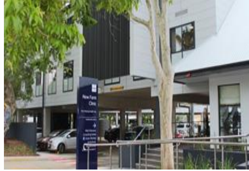
New Farm Clinic – 36 new beds and major refurbishment
