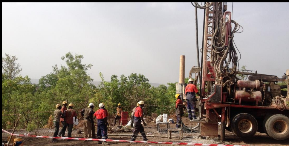
READILY ACCESSIBLE DRILL RIGS AND EQUIPMENT
