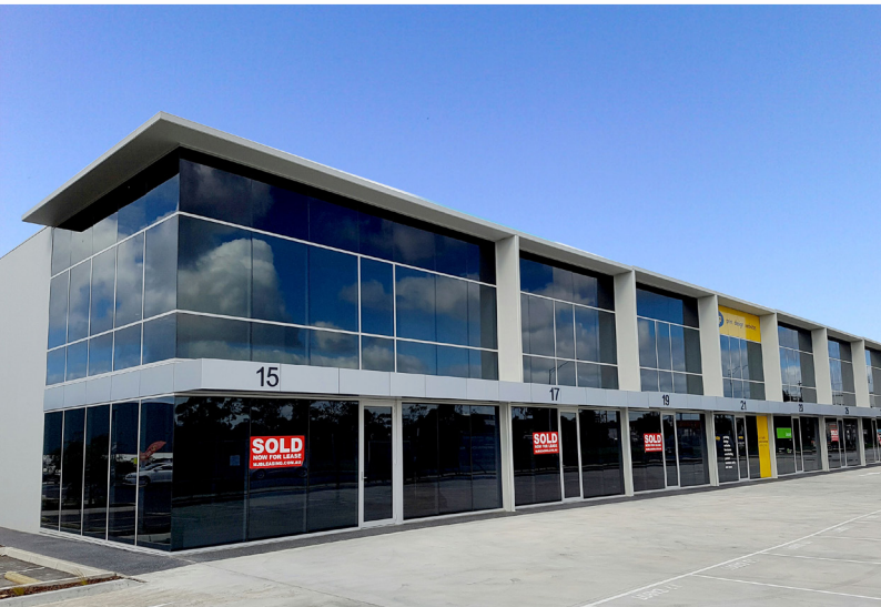
MILLERS JUNCTION BUSINESS - ALTONA NORTH, VIC FOLKESTONE AND WILMAC'S DEVELOPMENT
