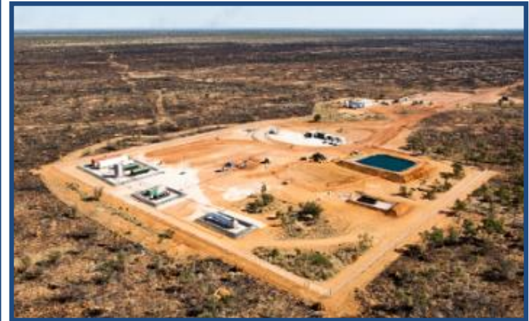
Ungani field facility
