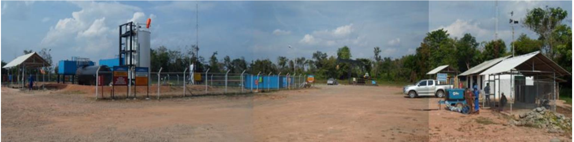
Bunian Central Production Facility
