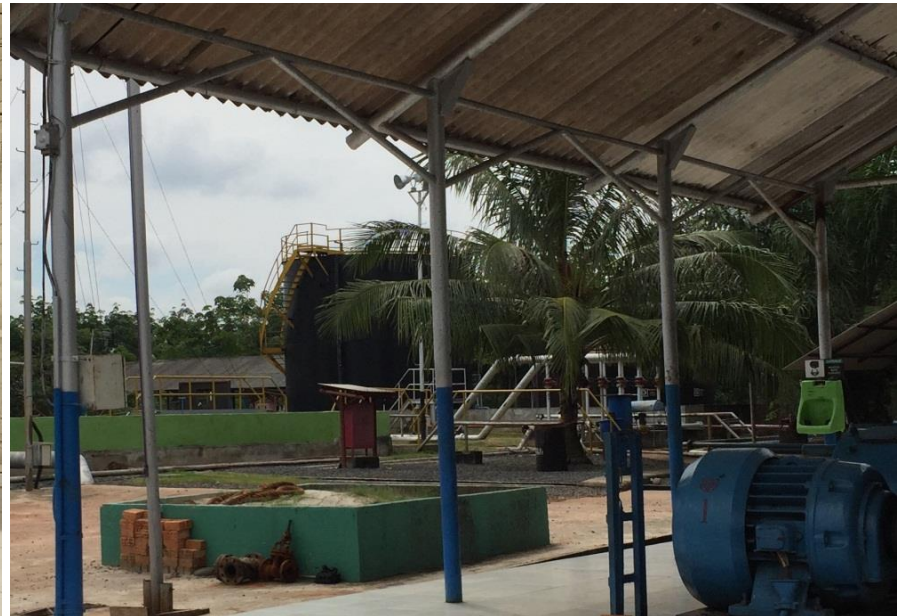
Talang Jimur Transfer Station
