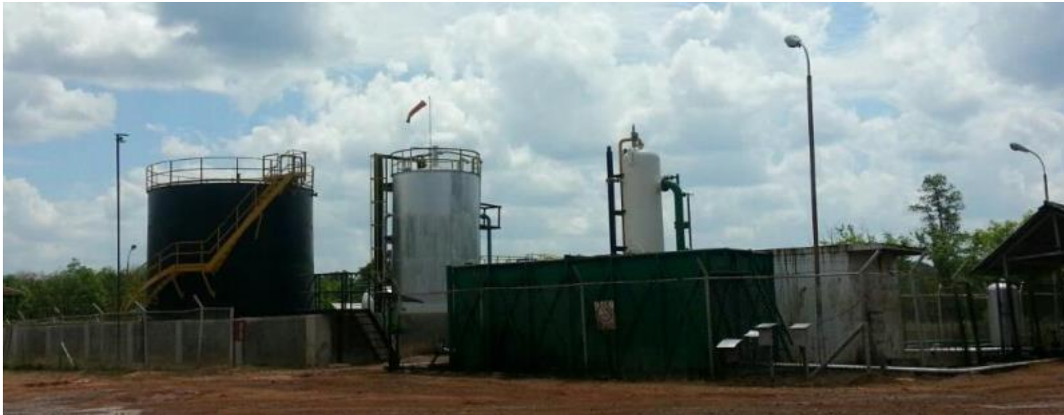
Bunian Central Production Facility
