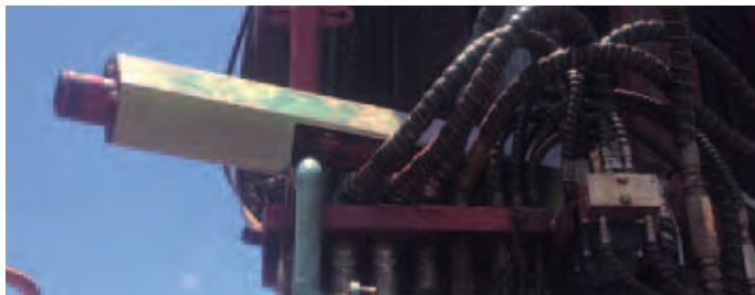
New scatter guard installed
