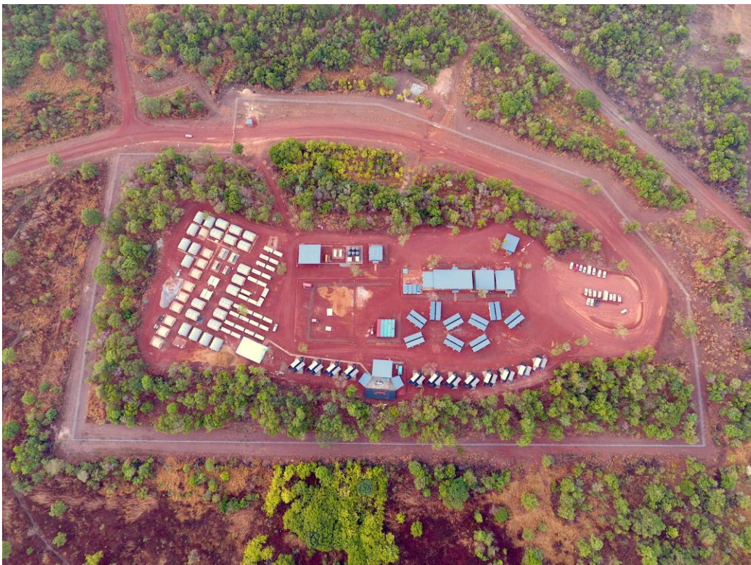
Photo 6: Aerial view of the Sissingué Camp nearing completion
