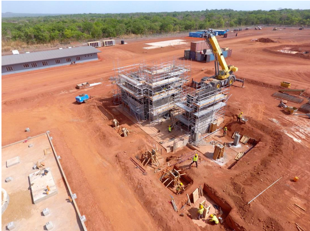
Photo 4: Foundations for SAG Mill well advanced
