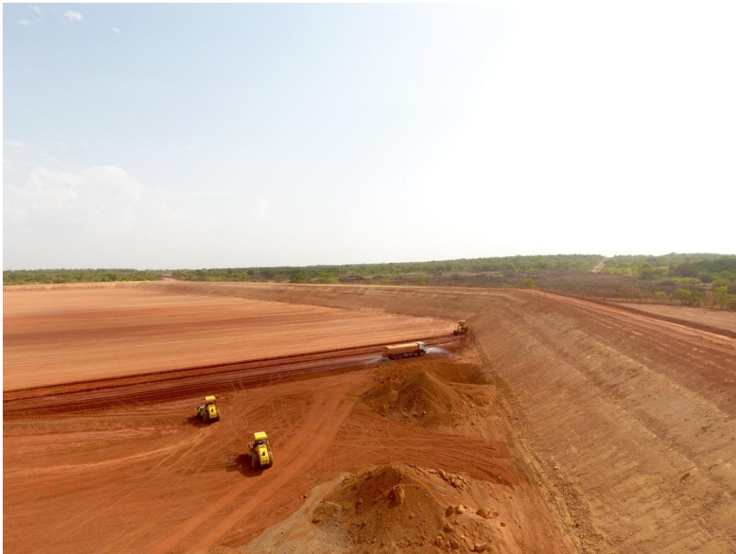
Photo 1: Tailings Dam construction showing compaction of dam floor
