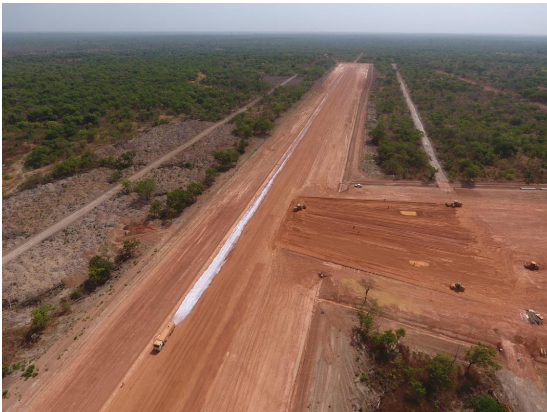
Photo 2: Sissingué's airstrip with sealant being applied
