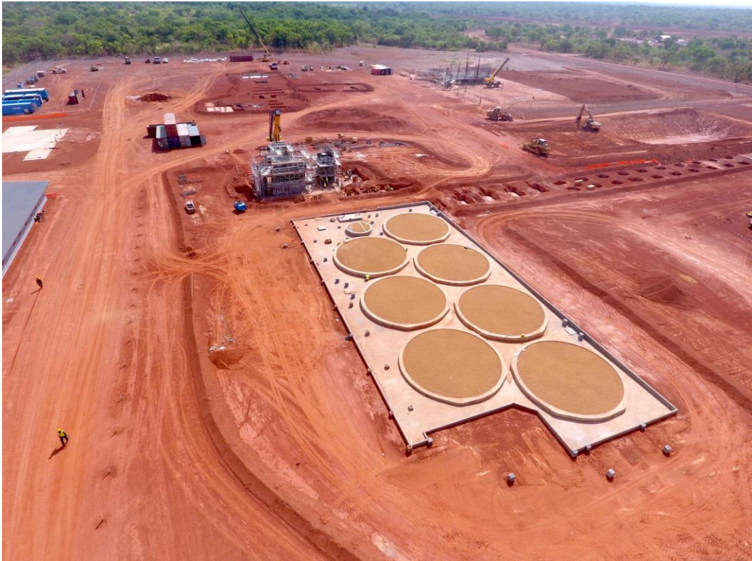
Photo 5: Foundations for the CIL tanks well advanced
