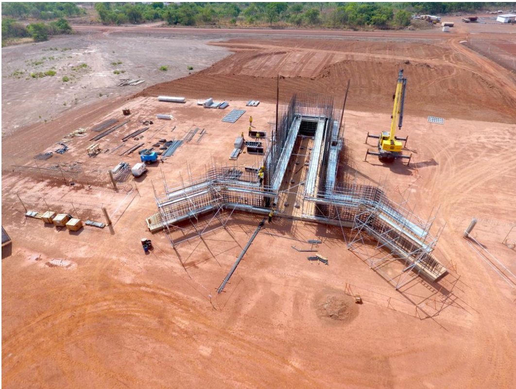
Photo 3: Formwork and reinforcing in place for Crusher foundations
