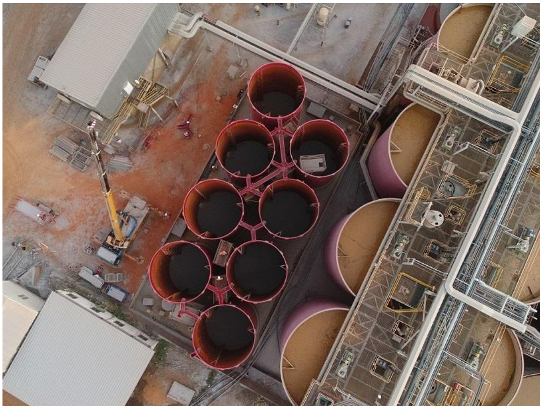
Figure 4: Syama Project 85 calcine CIL tanks installed
