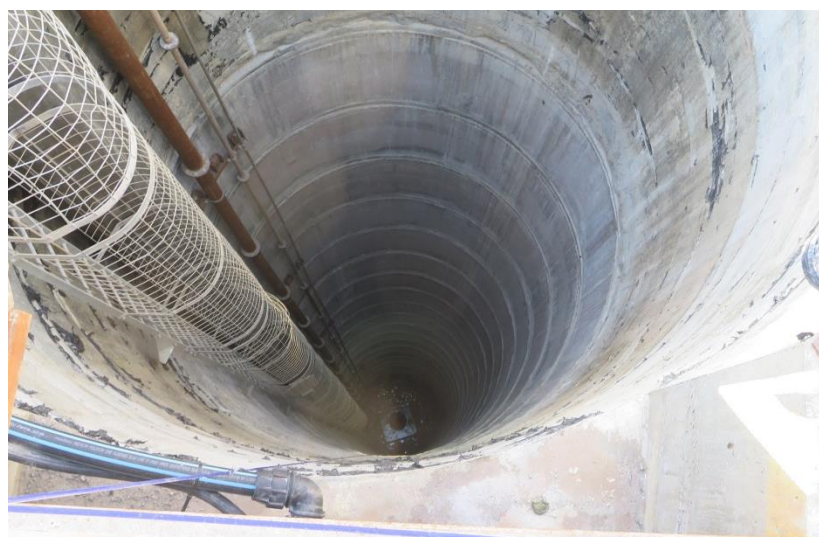
Ventilation shaft (raisebore) at Spotted Quoll
