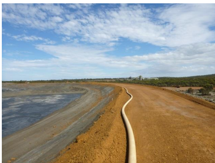
Cosmic Boy completed TSF 2.0m wall lift with discharge ring main being re-installed
