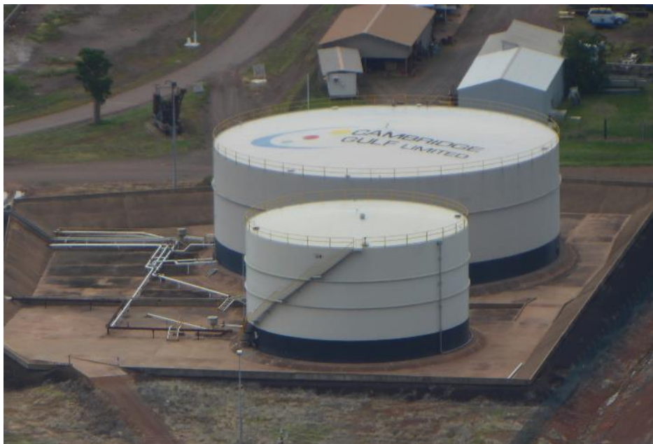
80,000 barrel and 30,000 barrel tanks at Wyndham
