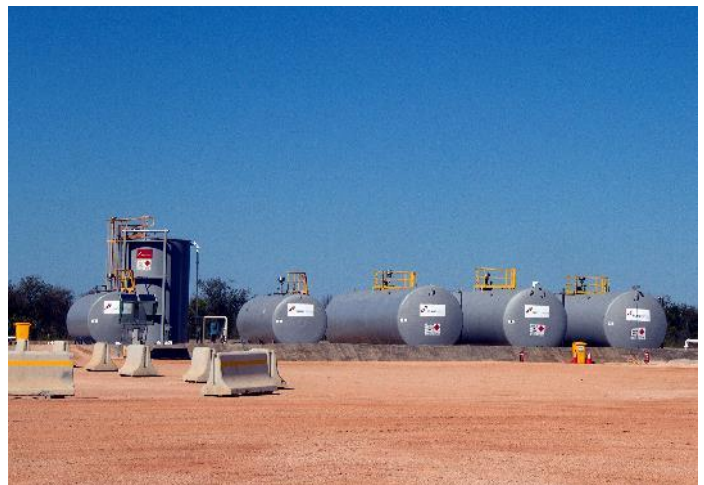
Ungani production tanks
