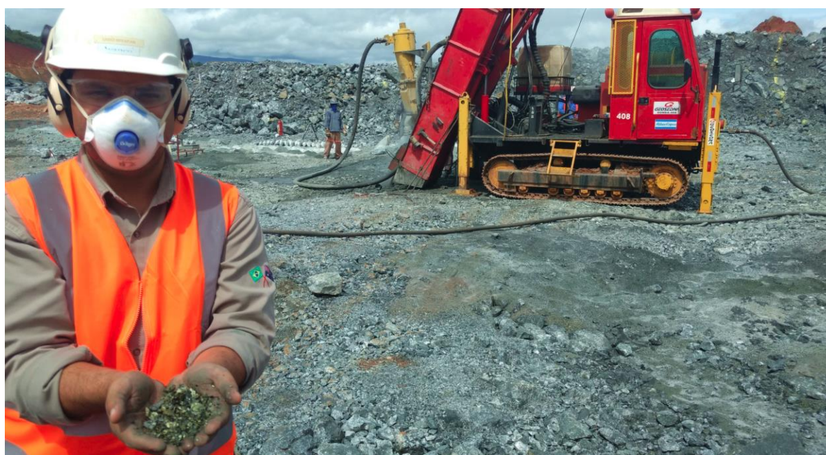
Grade Control Drilling in the Stage Two pit
