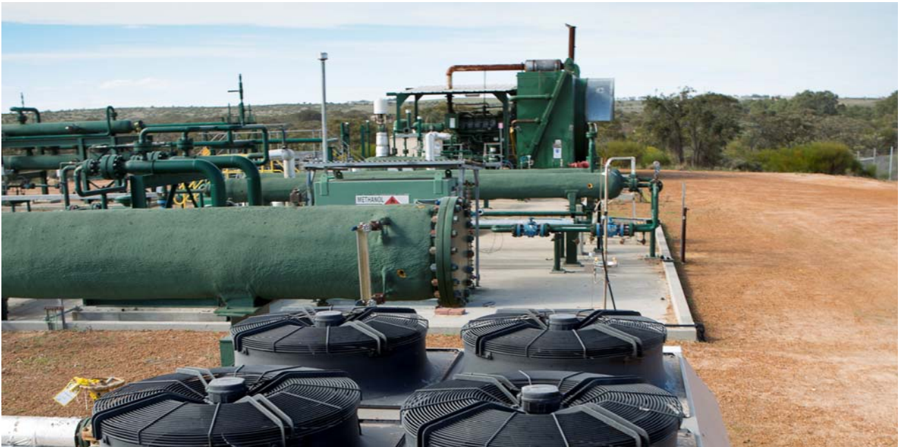
Above: Xyris Production Facility, Waitsia Stage 1A, northern Perth Basin
