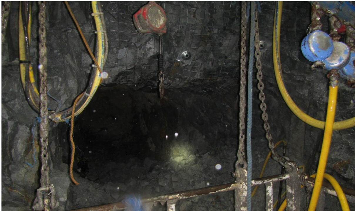
Photo 1: E15 sinking stage at the Level 3 break through
