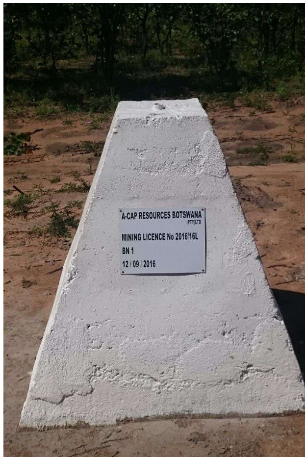
Beacon construction around the ML boundary
