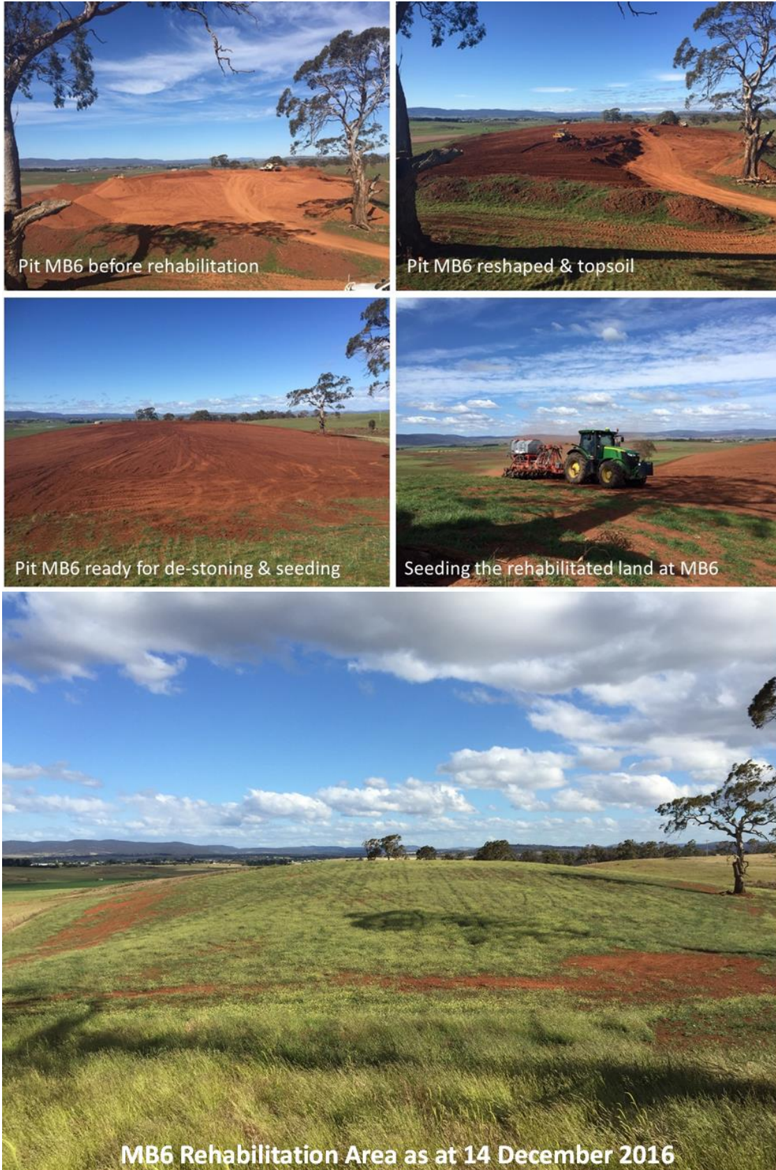
Figure 5: photographic record of rehabilitation processes, with Pit MB6 as the case study
