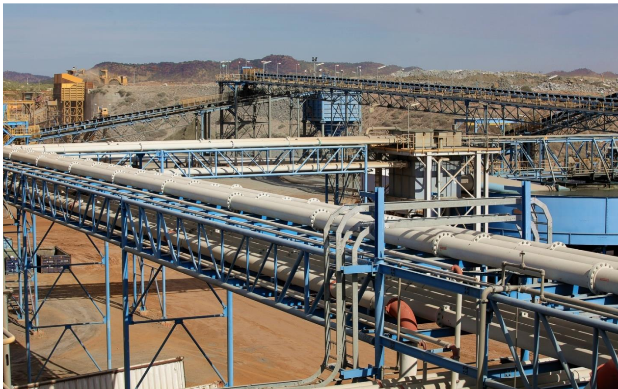
Figure 02: Looking towards the crushing circuit (left rear) and ROM (far distance) from the gravity jig area.
