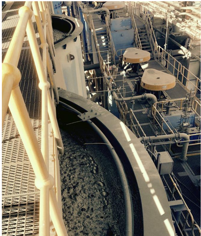
Figure 02: The Rocklands Process Plant includes 11 copper flotation cells including rougher, cleaner, cleaner scavenger and recleaner cells, that preferentially extract copper sulphide minerals to produce a sulphide copper concentrate via froth flotation techniques.
