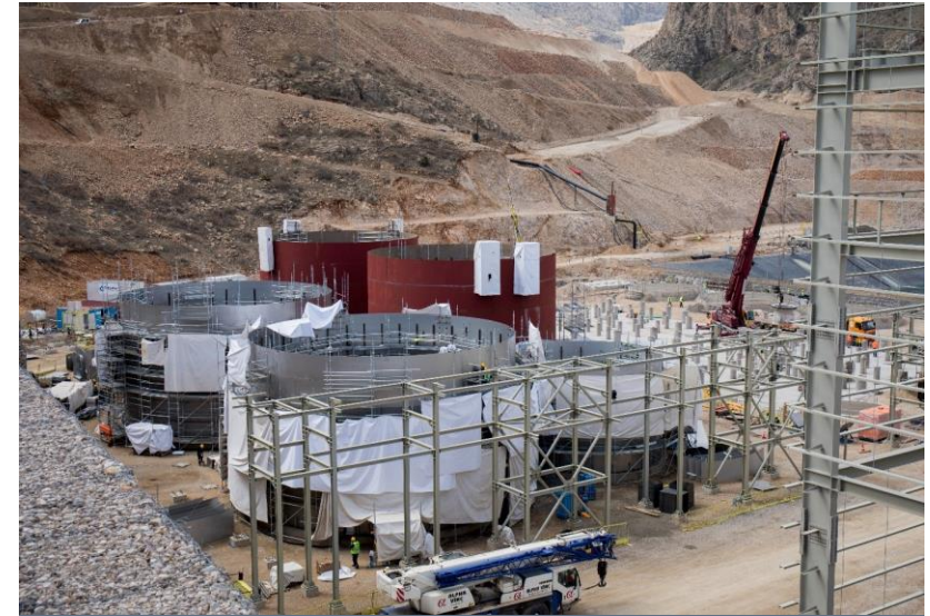
Acidulation Area, Decant & POX Feed Thickeners
