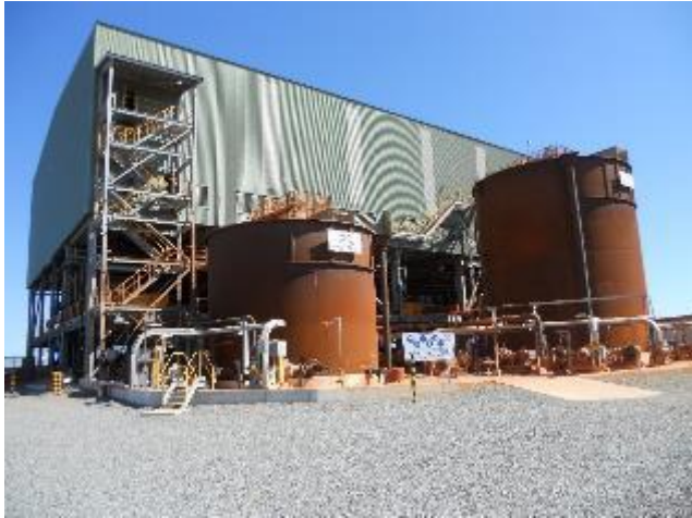
Press filtration building
