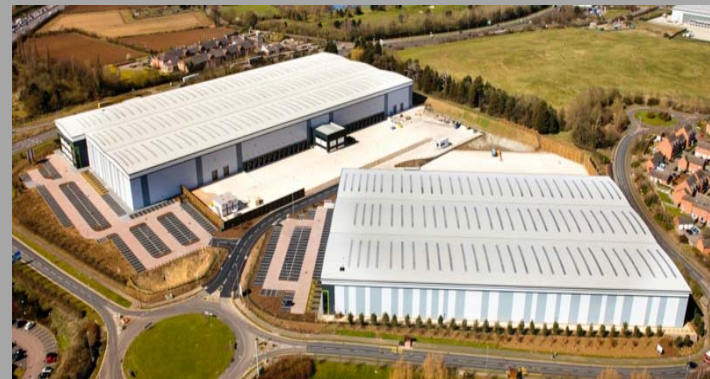
Northampton Commercial Park, Northampton
