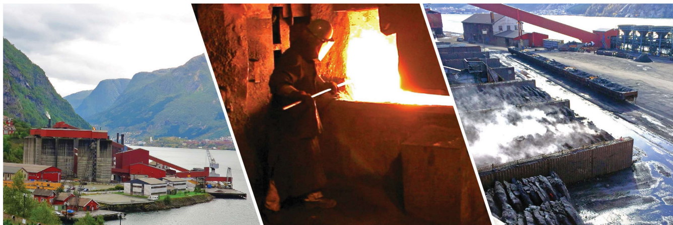
TiZir Titanium & Iron ilmenite upgrading facility, Tyssedal, Norway
