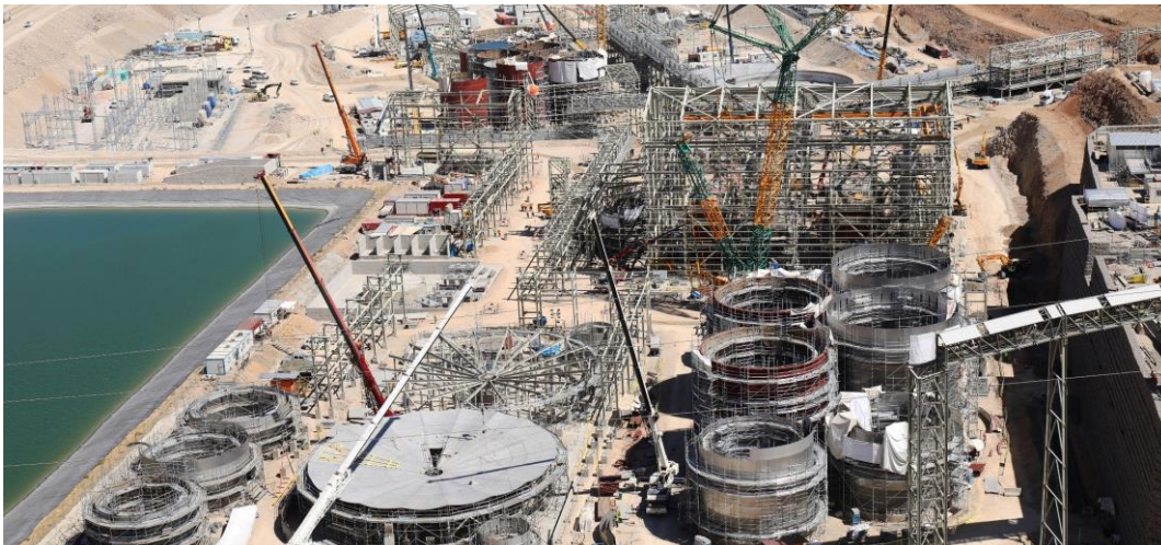
Iron Arsenic Precipitation, Acidulation & Autoclave Areas
