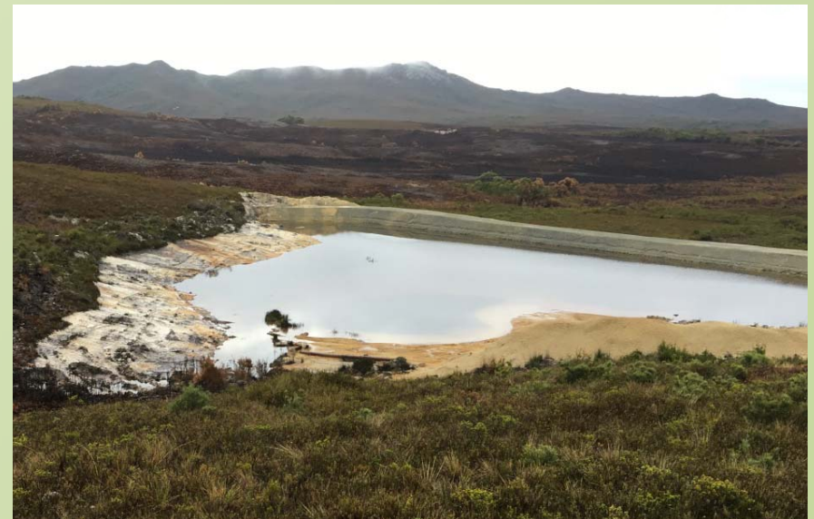
Existing Tailings Storage Facility at Granville Processing Plant
