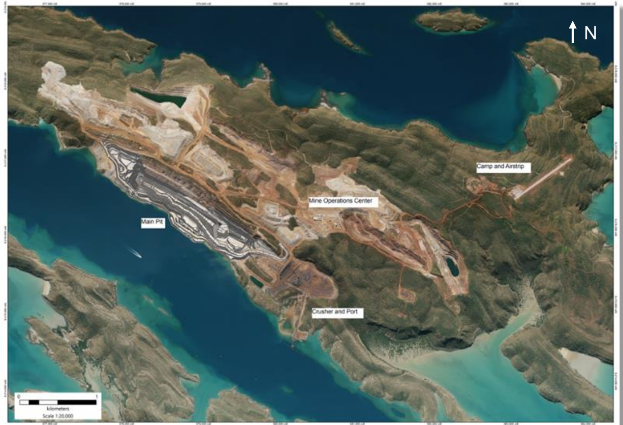
Koolan Island location and site layout showing Main Pit relative to existing site infrastructure, including crushing and port facilities, operations centre, accommodation camp and airstrip.
