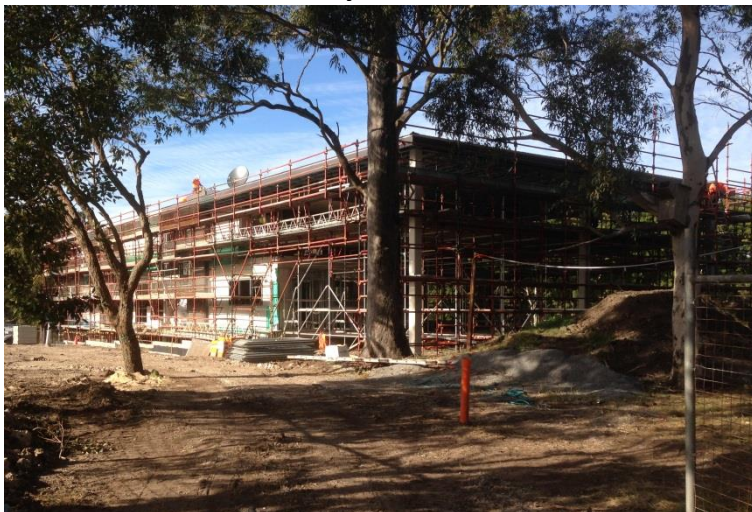
Newcastle – Community Centre under construction
