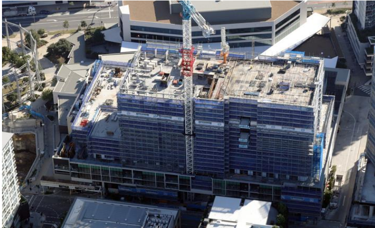
Newstead – 199 units under construction
