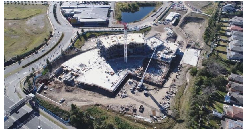
Bella Vista – 64 units under construction
