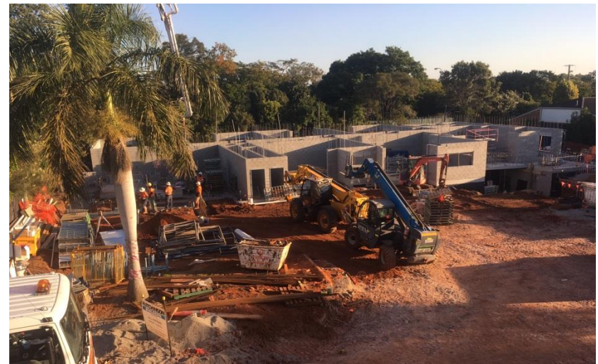
Robertson Park - 34 units under construction
