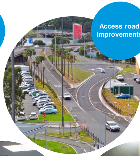
Terminal 1 expansion and improvements
