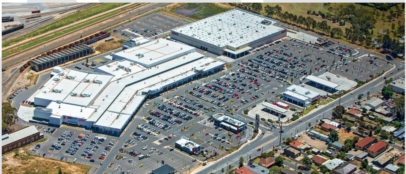
Churchill Centre North
