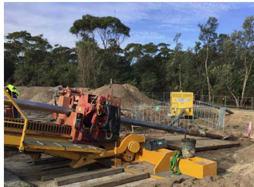
Horizontal directional drilling (HDD) in progress at Orbost
