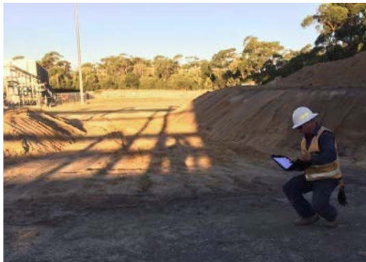
Bulk earthworks at Orbost
