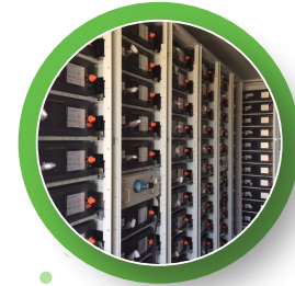
Western Power Perenjori Renewable Storage
