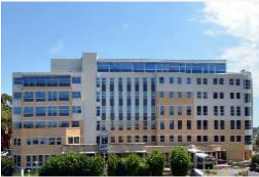
New accommodation wing at North Shore Private Hospital – 39 beds & theatres
