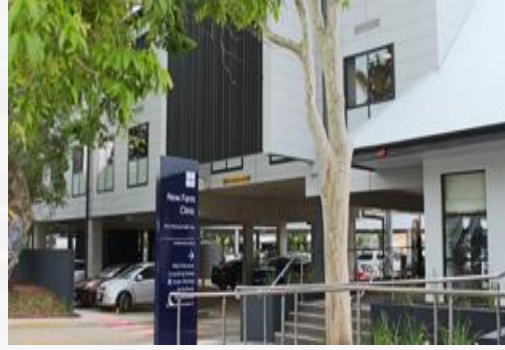
New Farm Clinic – 39 new beds and major refurbishment
