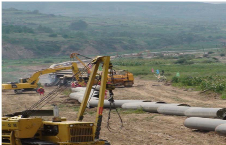
Gas and condensate export pipelines
