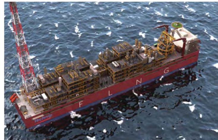
Near shore liquefaction facility
