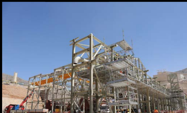
Pipe Rack & Piping Installation
