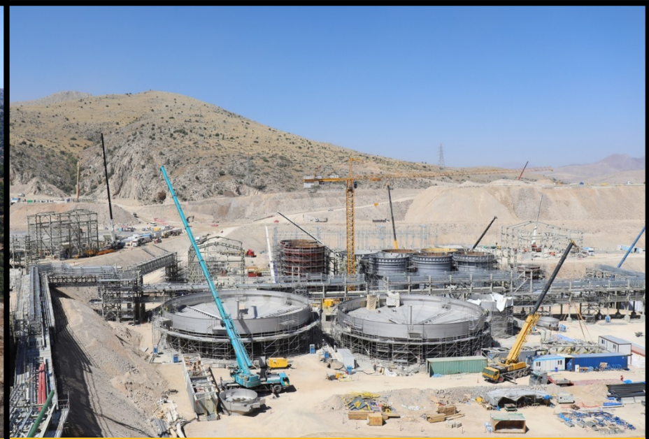
Counter Current Decantation (CCD) & Carbon-in-Pulp (CIP) Tanks
