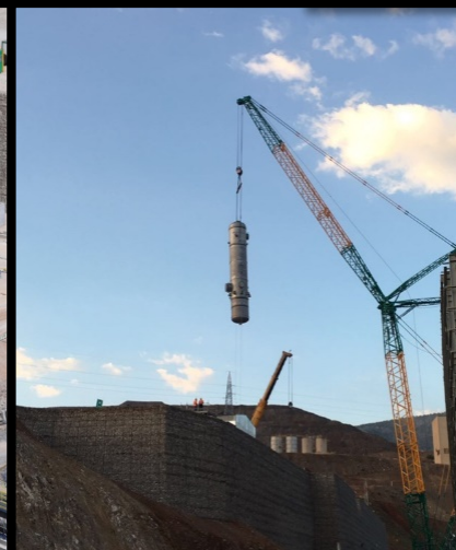
POX Heat Recovery Unit
