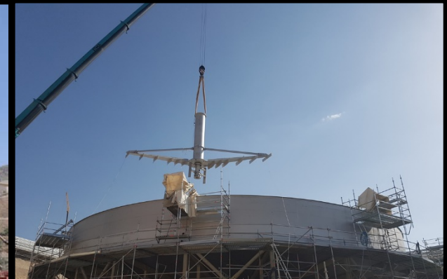
Thickener Rake Installation
