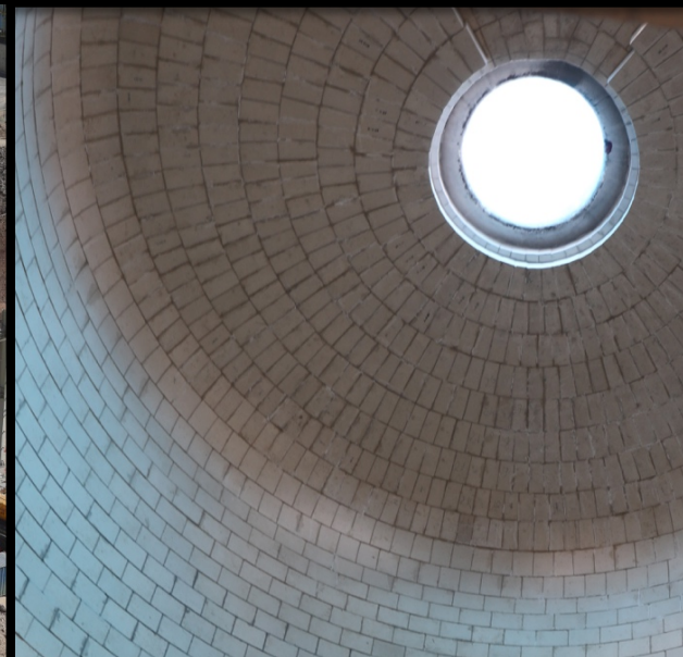
Flash Vessel (Brick Lining)
