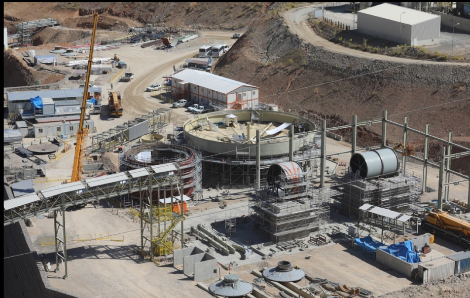
Grinding Area and SAG Mill Feed Conveyor
