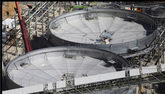
Feed and Decant Thickeners
