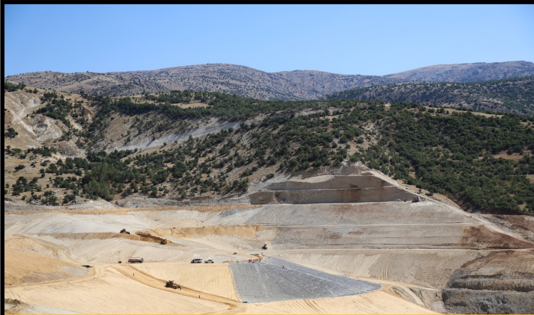
Tailings Storage Facility
