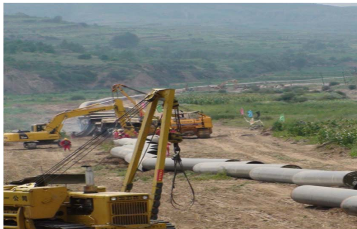
Gas and condensate export pipelines
