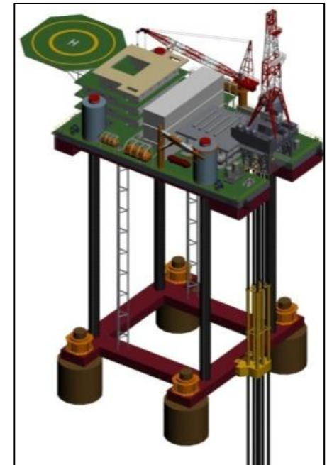
Leased mobile production platform (MOPU)
