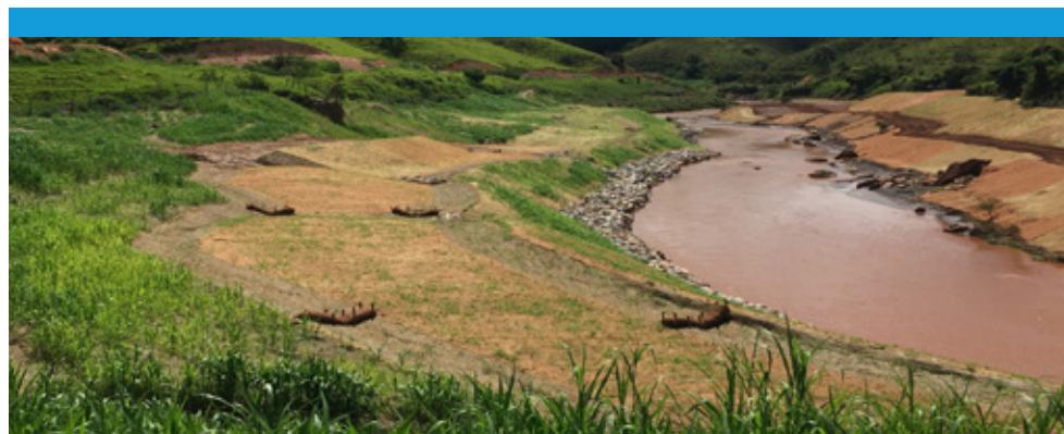
Remediation works along the Rio Gualaxo do Norte in the State of Minas Gerais.
