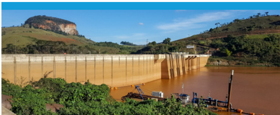
Candonga hydroelectric dam, the site of significant remediation works.
