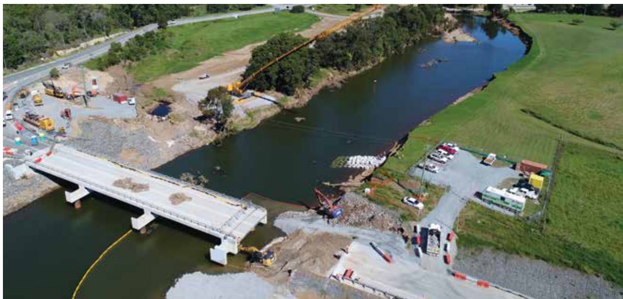
John Muntz causeway remedial works underway
