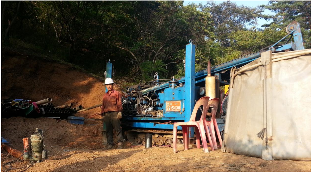
Photo 1: Diamond drilling rig set-up on drillhole UBD0002, testing Taipan and Cobra Targets, looking east
