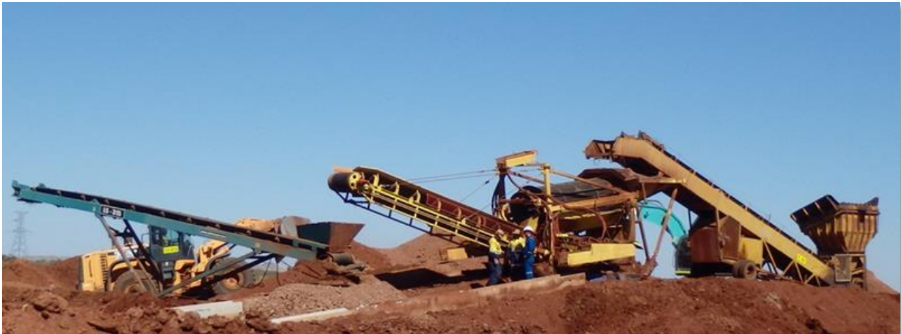
Figure 8: Nickol River gold processing plant
